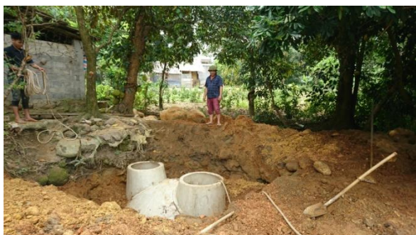
Photo 9: Installation of biogas
